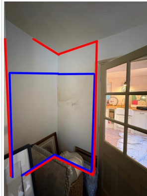
Blue = elevated moisture readings obtained
